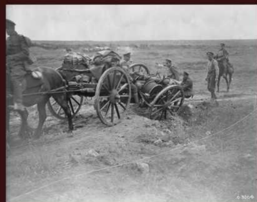
Canadian Signal Section laying cable. Advance East of Arras. Sept 1918. Library and Archives Canada MIKAN 3405814
