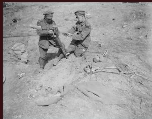
Canadian Signallers using German rifle as telephone pole, advance east of Arras, Sept 1918. Library and Archives Canada MIKAN 3405816
